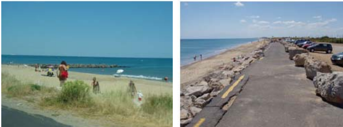
Figure 3 - Hard defence works: the groyne at the Castellias campsite, a rock seawall reinforcing the coastal road (from Gomboa et al., 2004).
